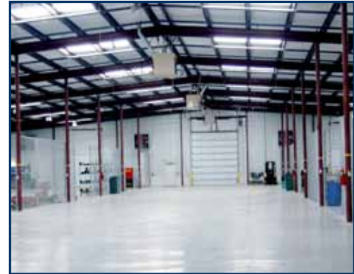
The Town of Louisburg utility departments moved from a building circa 1906, to this newly renovated 55,000-sq. ft. facility.
